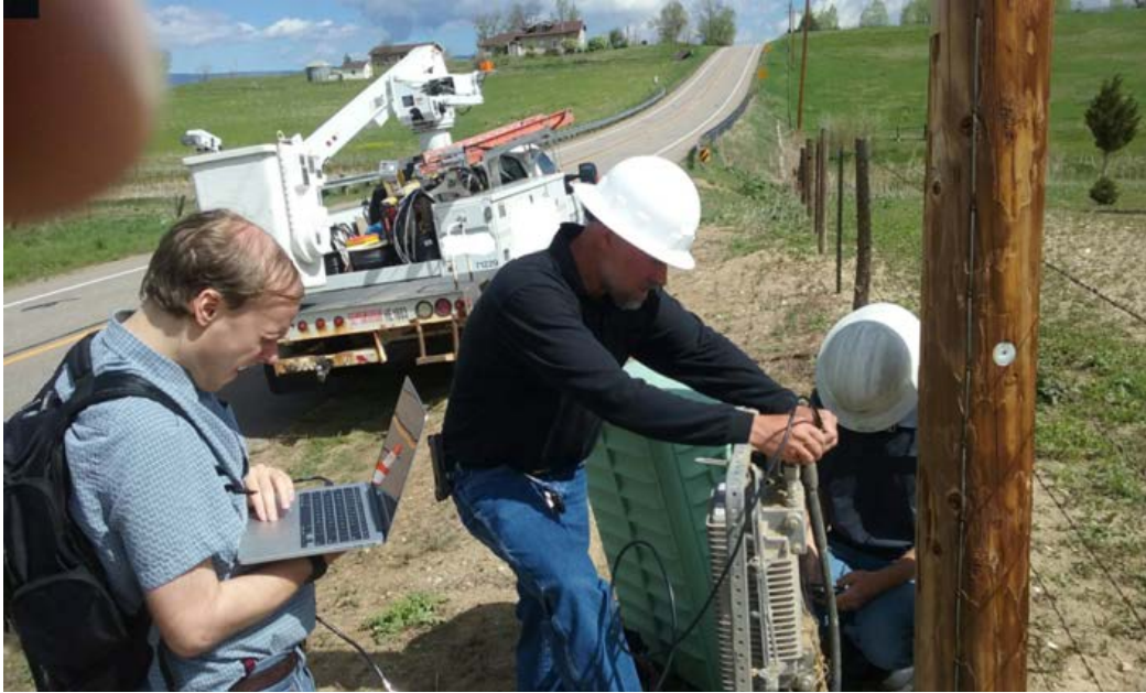
Figure VIII-4 - A Cablelabs Engineer Making a TDR Measurement in the Field. The SDR is in his Backpack
